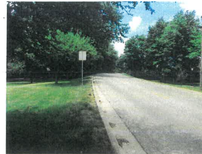
Observing sight distance looking north along 1st Street.
