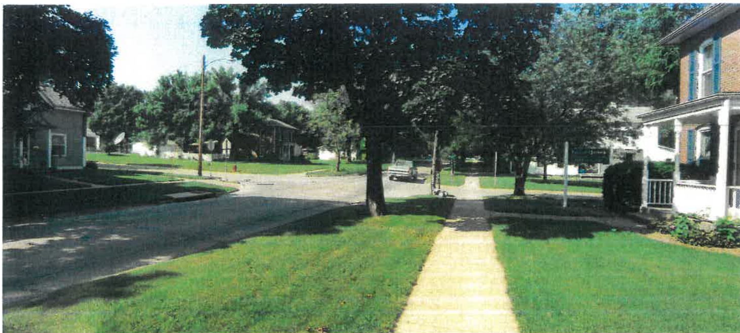
Looking north along Highway 1 near 4th Street at the existing site conditions.
