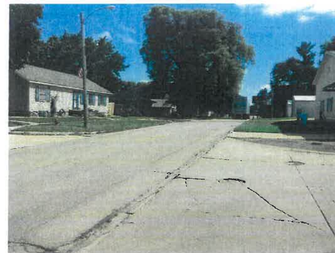
Observing sight distance looking north along Highway 1.
