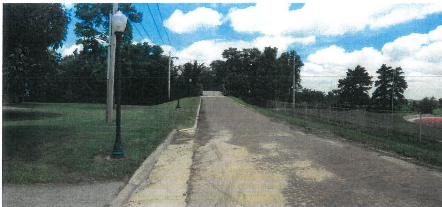
Existing conditions in Prairie Park along the Old Lincoln Highway.
