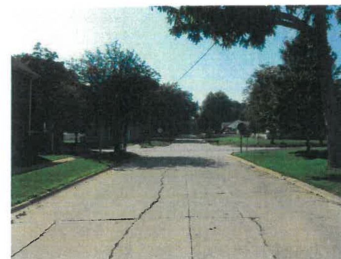
Looking west on 4th Street at the existing conditions of the intersection with Highway 1.
