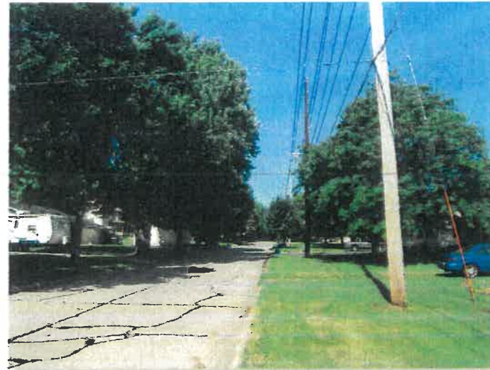
Existing curbside conditions looking west along 8th Street.
