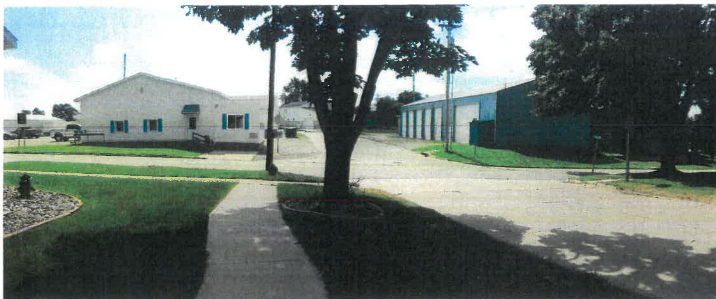
Existing conditions looking east at the intersection of Highway 1 and 7th Street.
