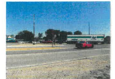
Intersection of Hwy 30 and Hwy 1. Source: Robin Hamadani
