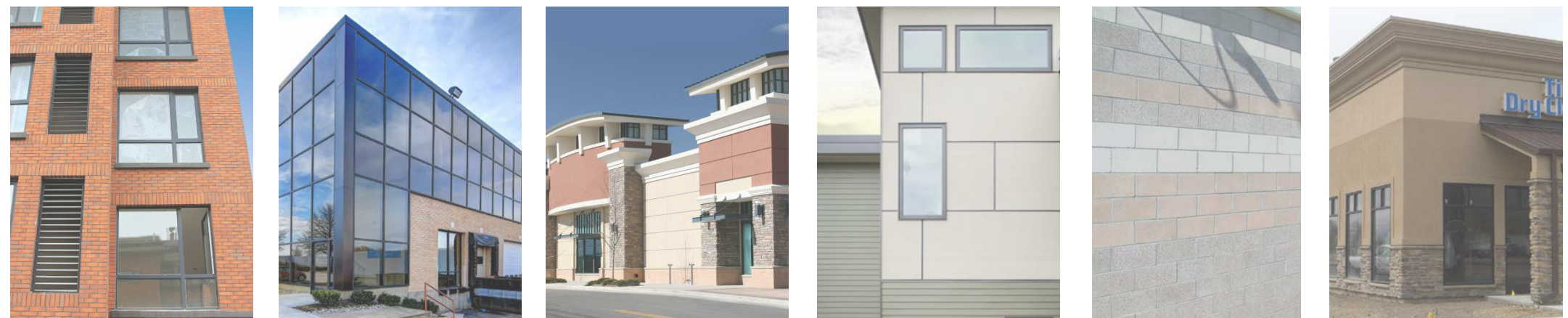
[ Building Materials Left to Right – Class A Brick, Class A Glass, Class C EIFs, Class C Fiber Cement, Class B Burnished Block, Class B Stucco ]
