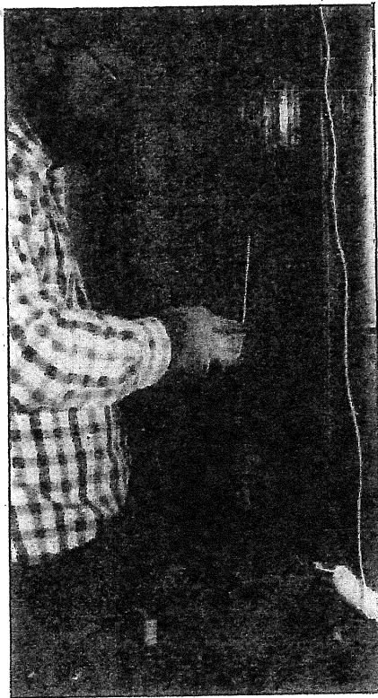
Maintaining a historic window may include work as basic as replacing a sash cord.
